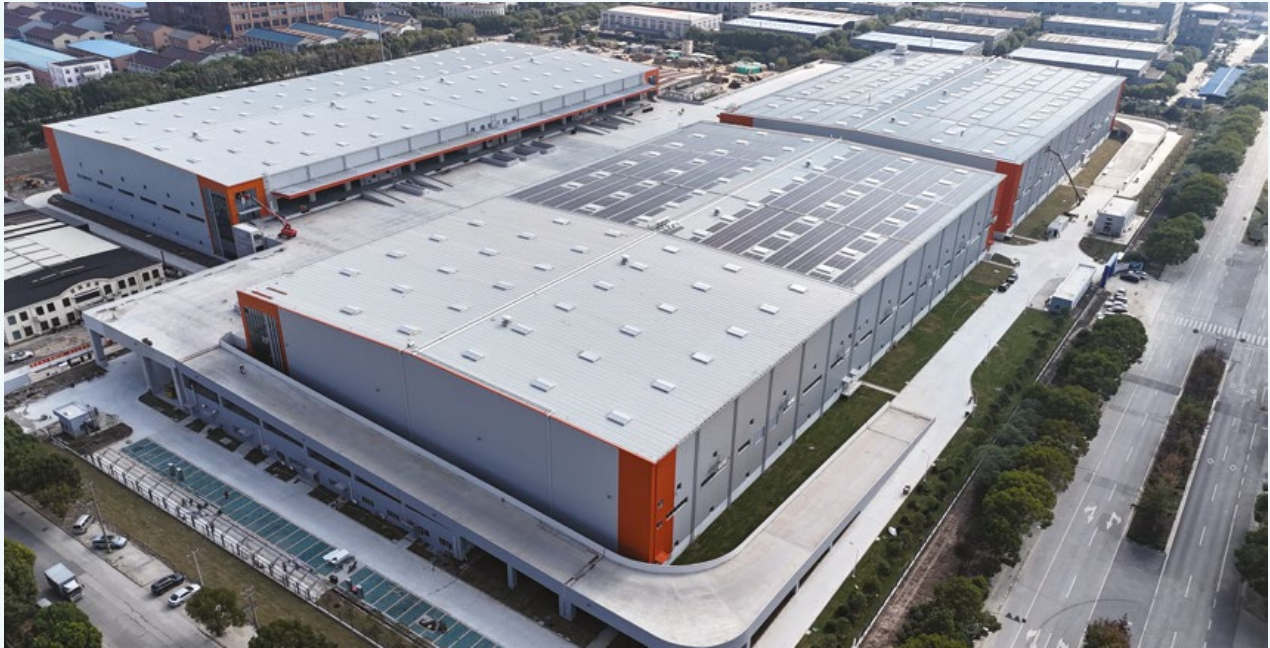
Mapletree Shanghai Fengxian Logistics Park is located in Shanghai, China.
