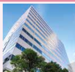
Omori Prime Building
