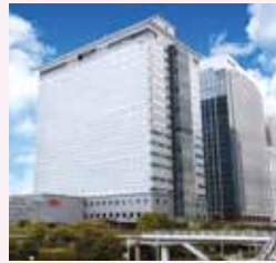
Fujitsu Makuhari Building
